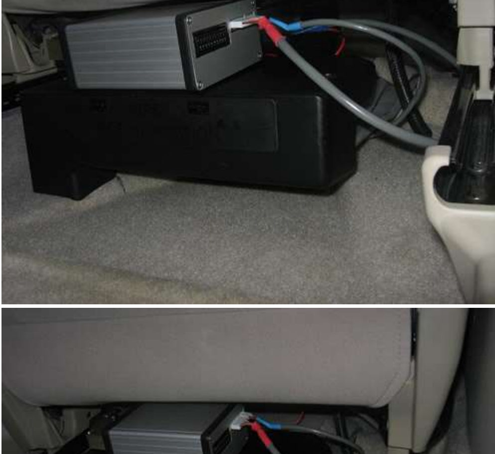
7) CAN-View Molex cables connected on inboard side Just another viewpoint to show the other side.
