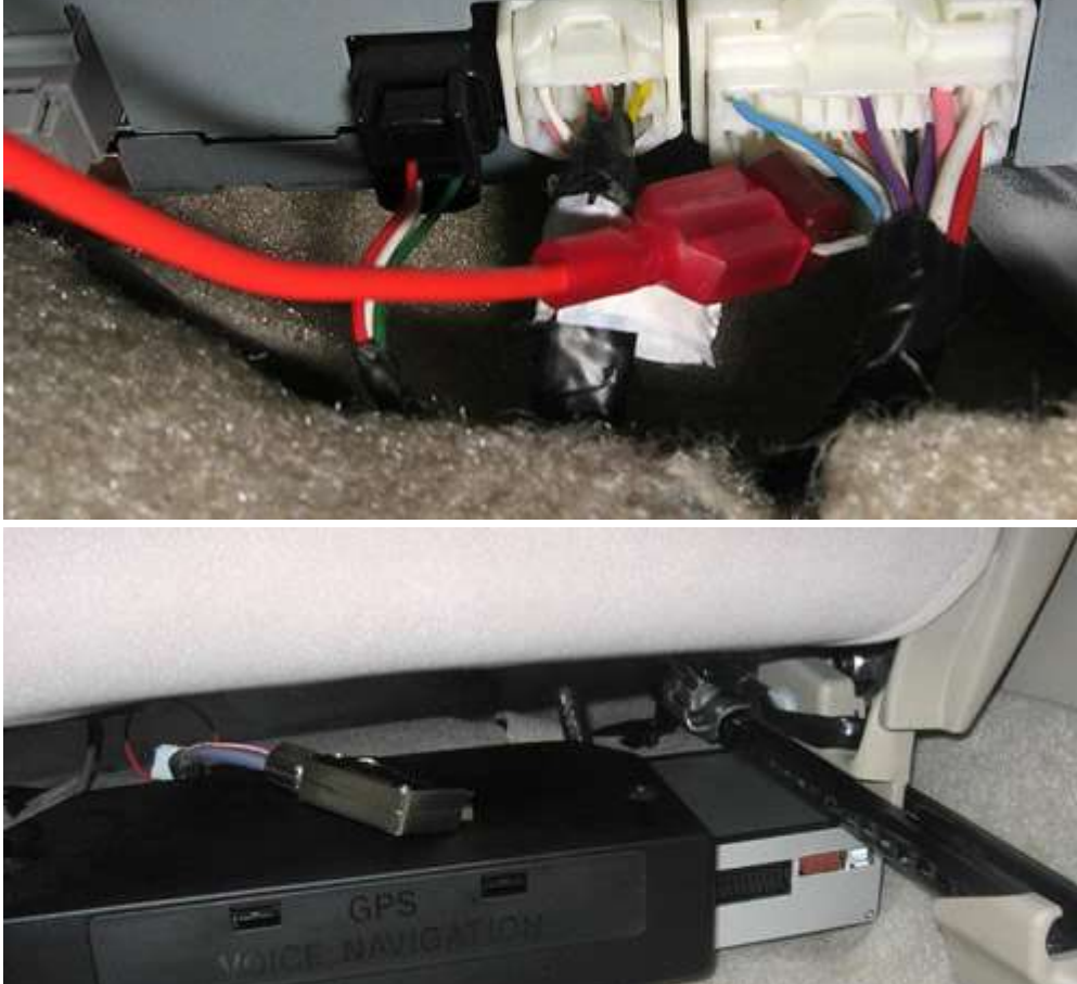
3) Tap installed on grey wire on plug N2 of NAV unit and red spade terminal of CAN-view cable 1 inserted firmly into tap.
